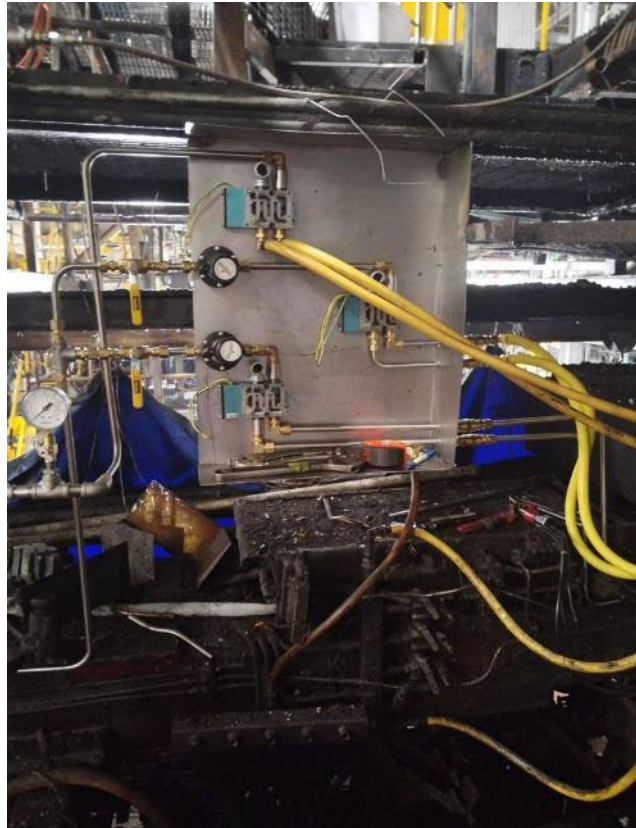
Hoses and pipes are installed
