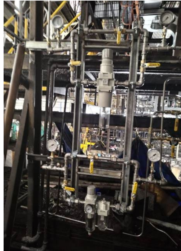
Air By-Passes are installed and connected
