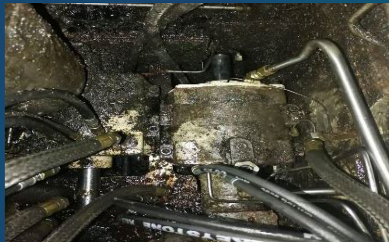
Corrected installed cover
